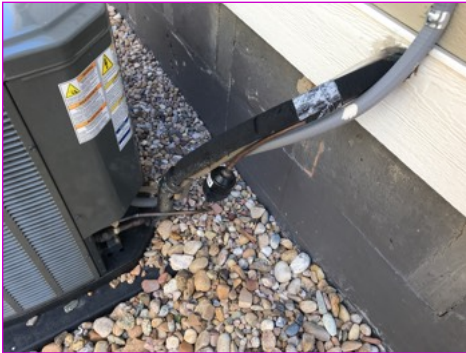
CENTRAL AIR CONDITIONER AC Refrigerant Lines
