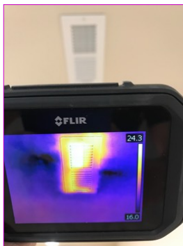
FURNACE Furnace Operation
